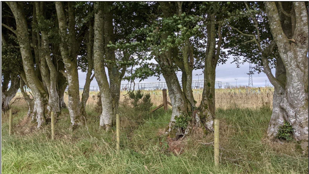
Photo 2: Western Site Boundary Embankment with Rothienorman Substation Beyond
